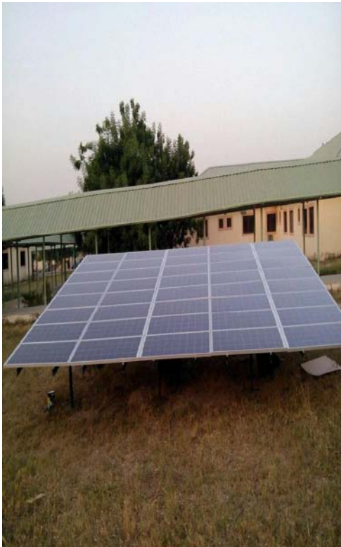
3kW solar PV mimi-grid in Talasse General Hospital, Balanga LGA, Gombe State (2013)
